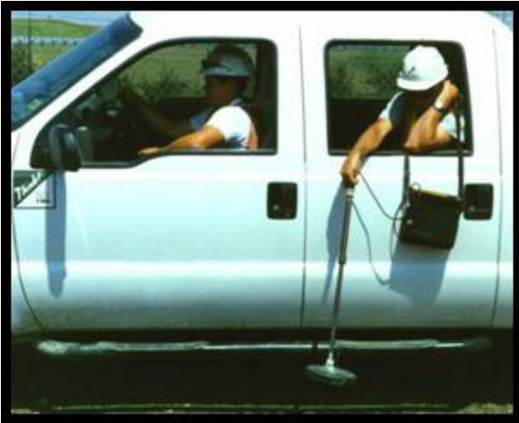
Drive the Duct Path
